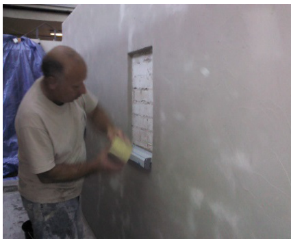
Mortar Application on Wall
