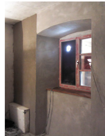
Final result of Window Mortar
