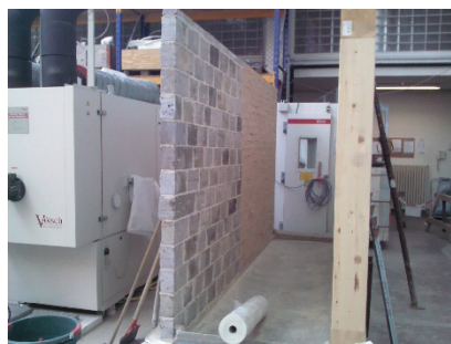
Stone and Brick Wall
