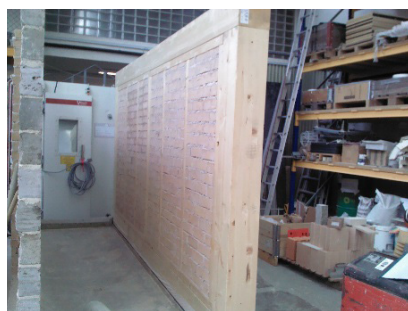
Wood Timber Wall
